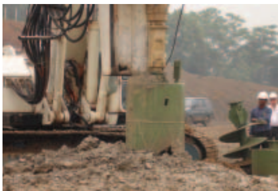
Boring to install the 30" conductors
