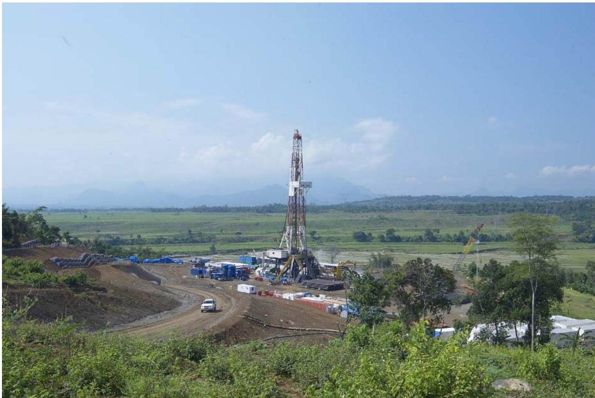
Great Wall Rig 93 drilling Pasundan-1 exploration well
